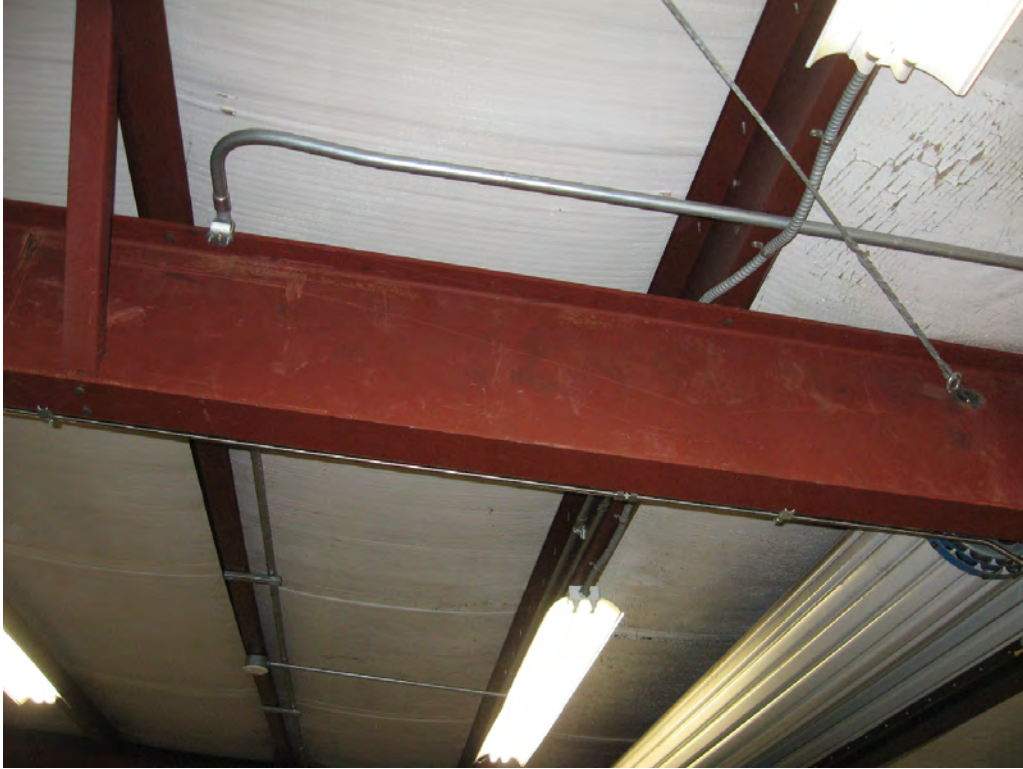
Figure 36: A new Avigilon security camera will be mounted at this ceiling location to monitor the Kelly Building door on the south elevation.
