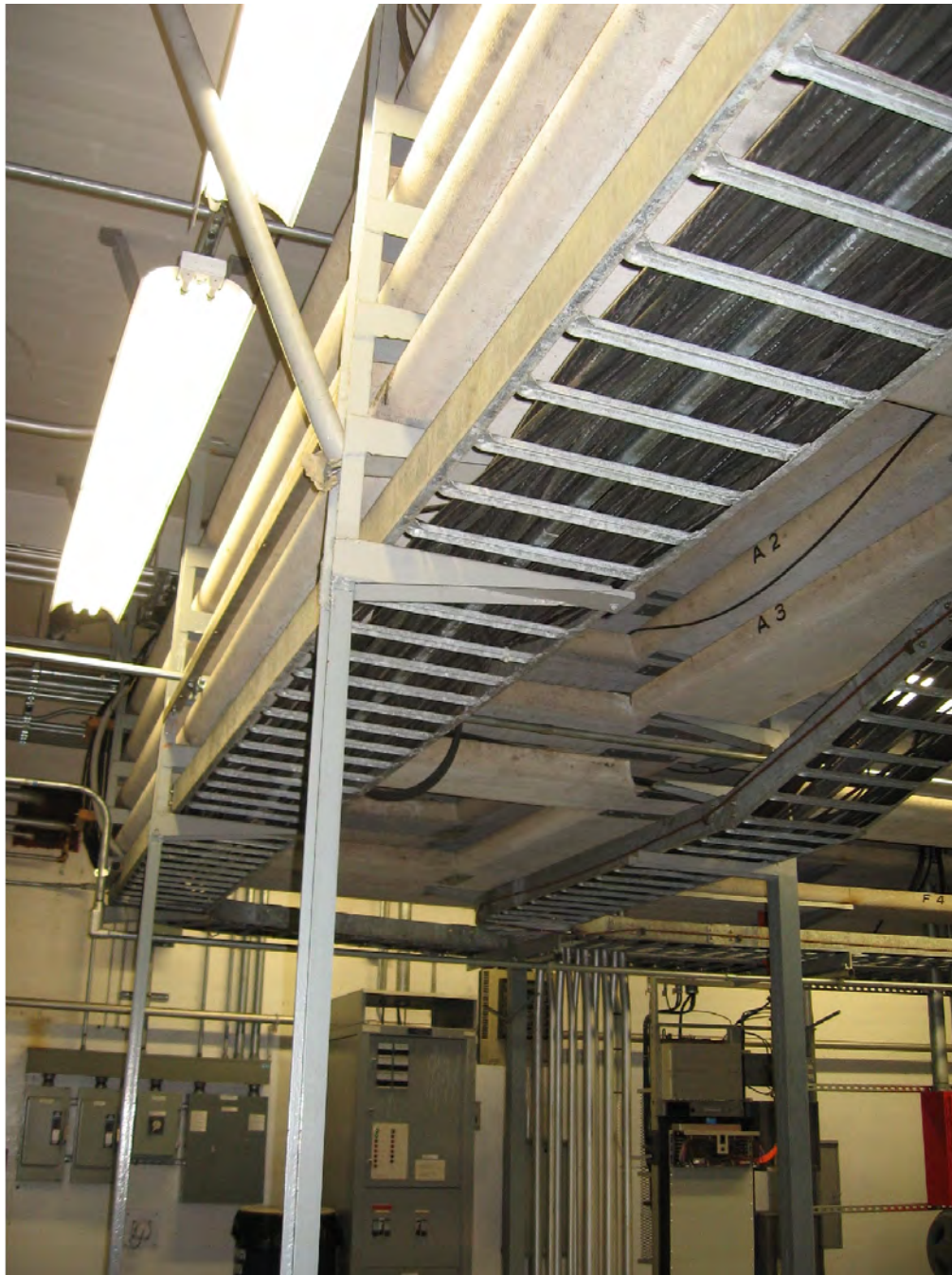
Figure 51: The location for the proposed Avigilon camera for the northeast door would be on the underside or side of the ca. 1990 metal cable trays in the Spreading Room.
