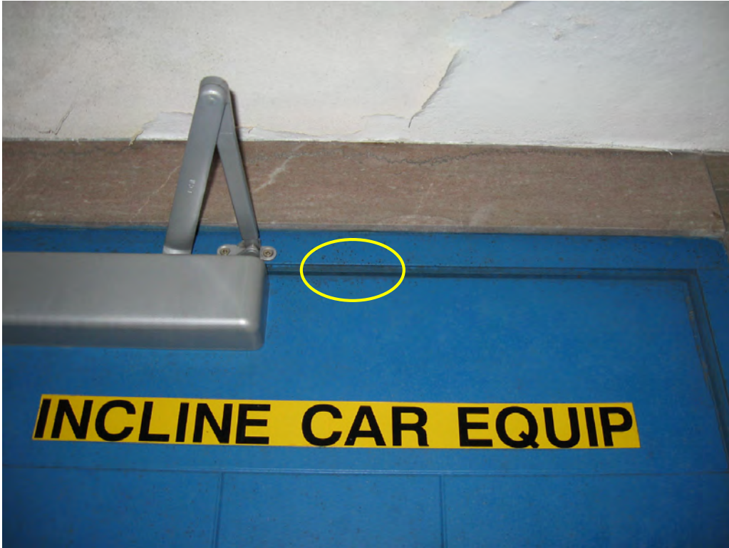
Figure 47: The location of the proposed PIR sensor on the interior of the Incline Car Room door is shown as the yellow circle.
