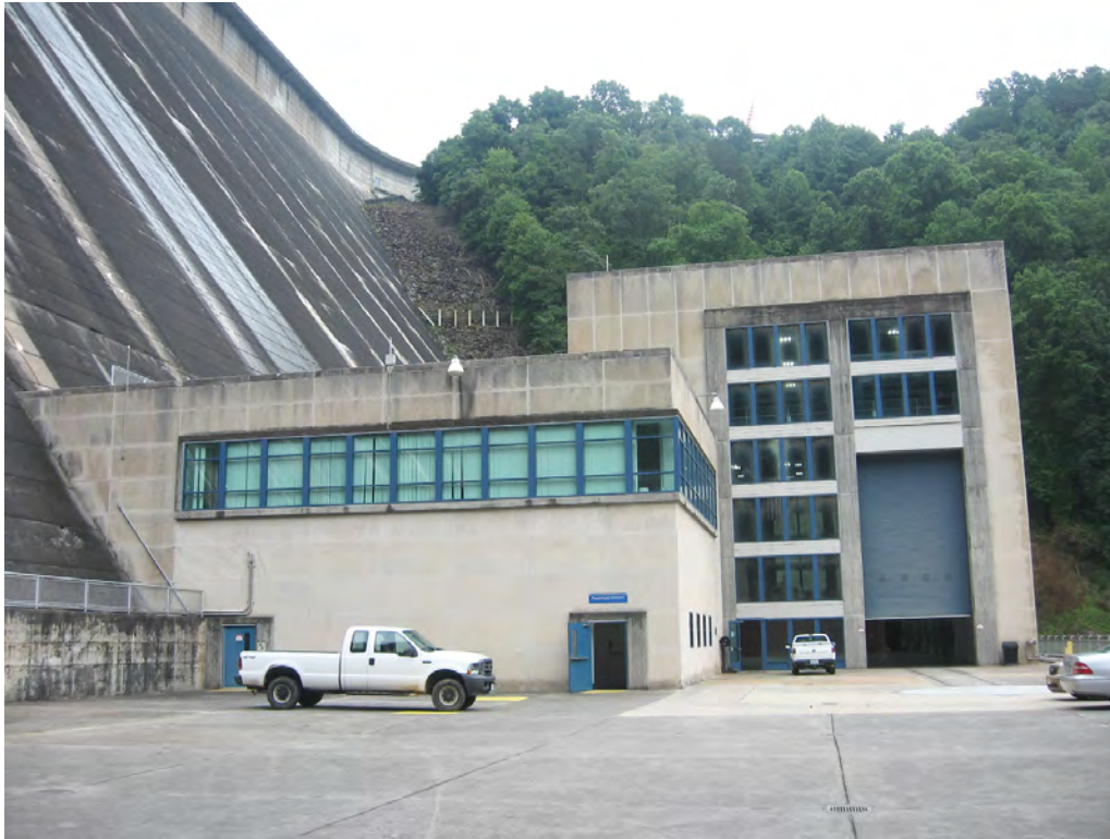
Figure 3: Fontana Powerhouse, west elevation.
