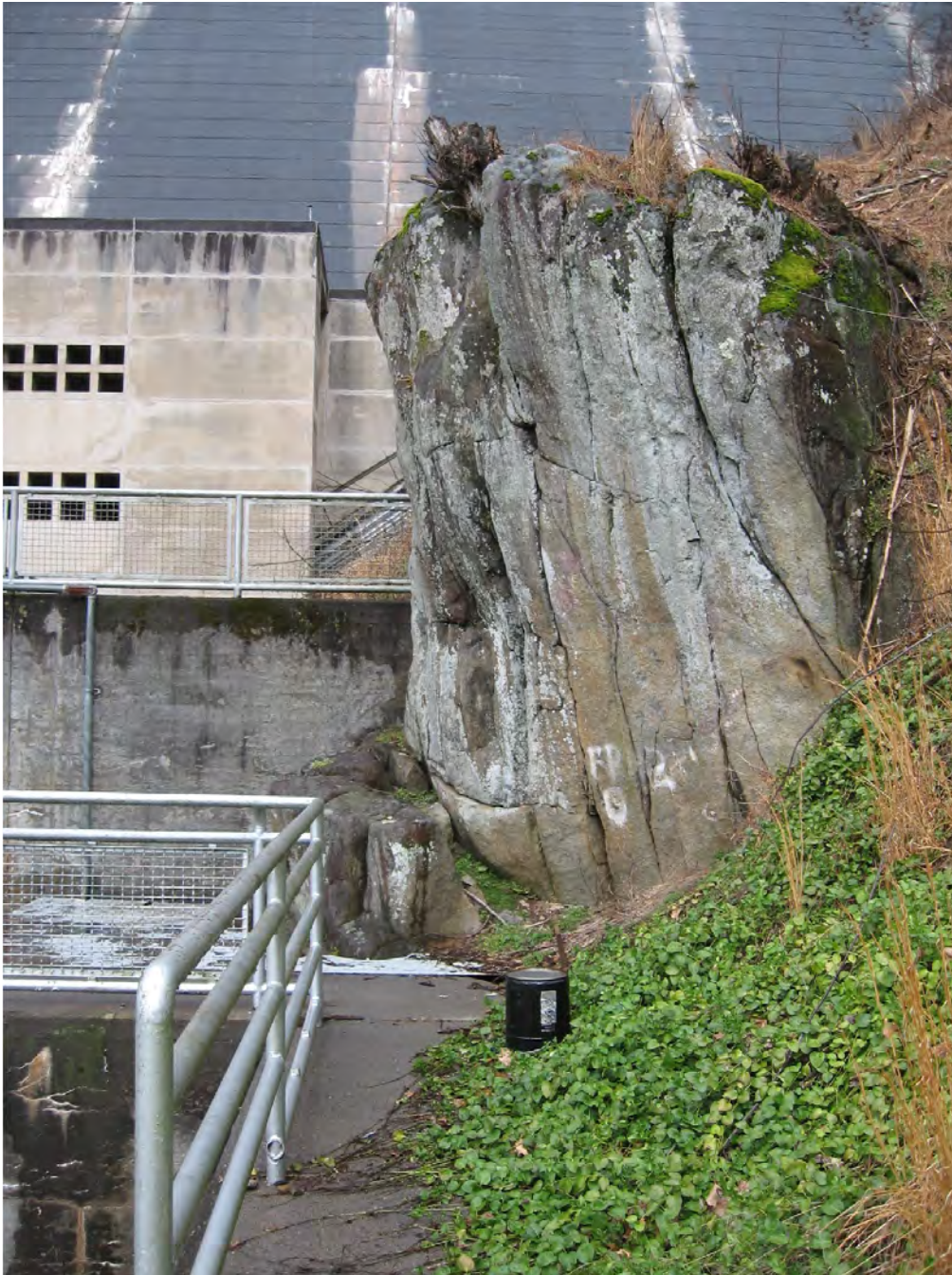
Figure 69: View of the existing fence on the east side of the powerhouse. A new seven-foot high chain link fence and security gate will be added at this location.
