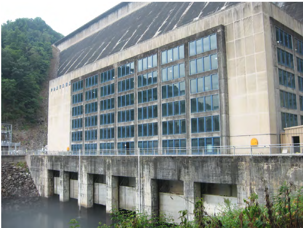
Figure 4: Fontana Powerhouse, south elevation.
