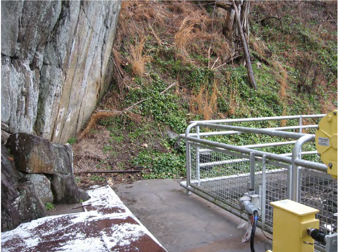
Figure 68: This area on the east side of the powerhouse will be fenced with a new seven-foot high chain link and barbed wire fence with a pedestrian gate. This view is to the southeast.
