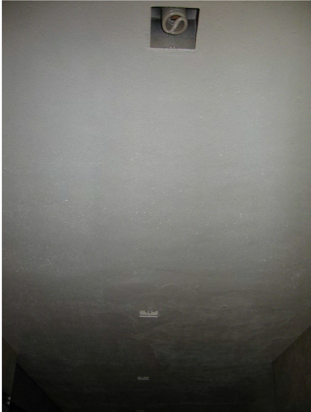
Figure 30: A new Avigilon security camera will be added to the ceiling inside the northwest Powerhouse door entrance.
