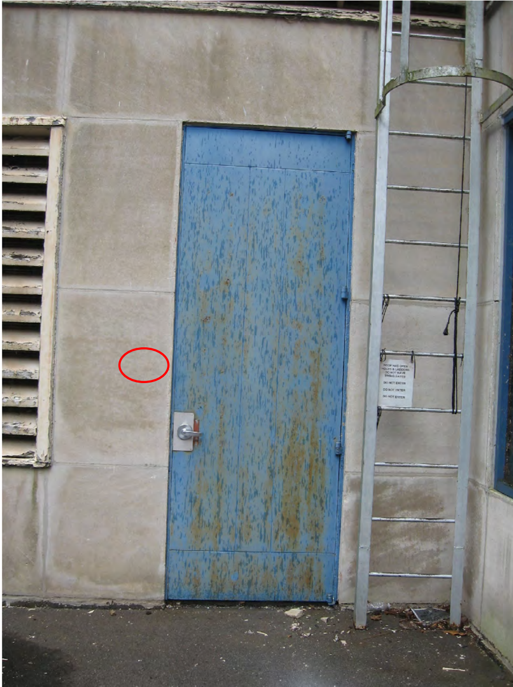
Figure 31: A security card reader will be added to this location circled in red adjacent to the upper rear deck door. This door is within the recessed bay on the north elevation.
