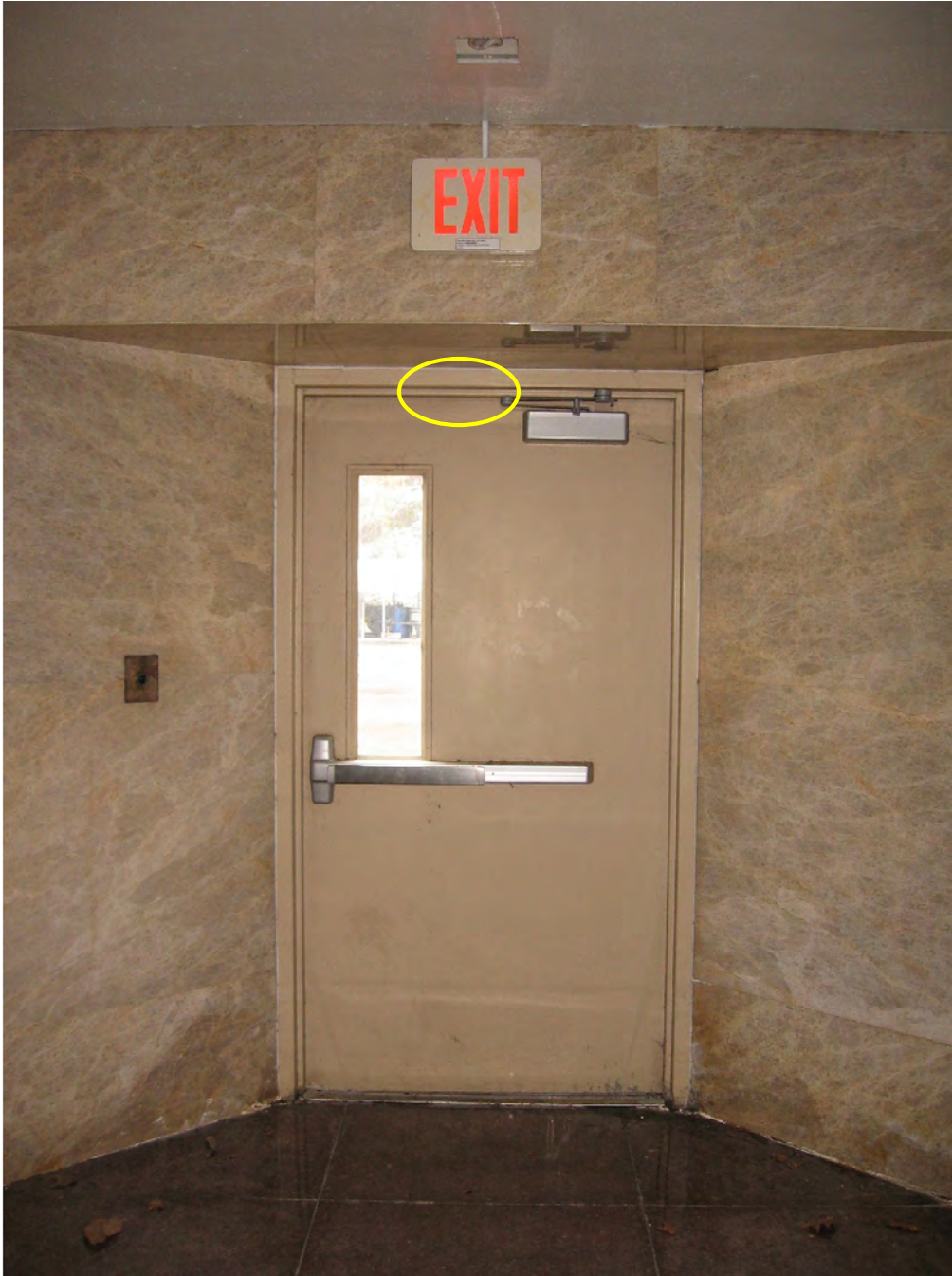
Figure 29: This view is of the interior of the northwest Powerhouse door. The location of the passive infrared sensor (PIR) is shown as the yellow circle.
