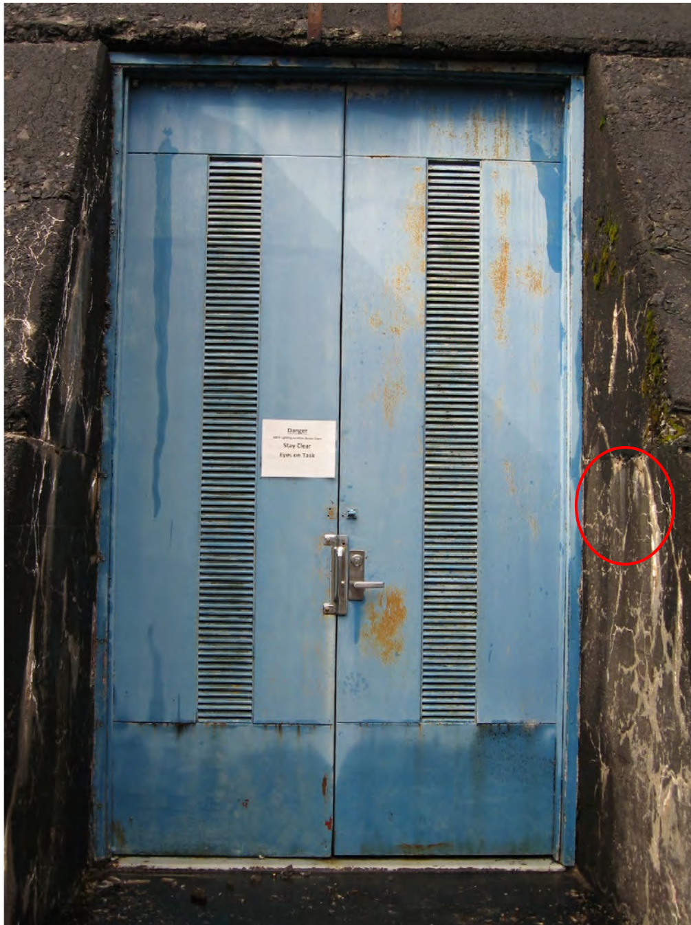
Figure 39: A new card reader will be added to this location circled in red adjacent to the entrance to the west-end Head Gate Gallery door on the south elevation of the dam.
