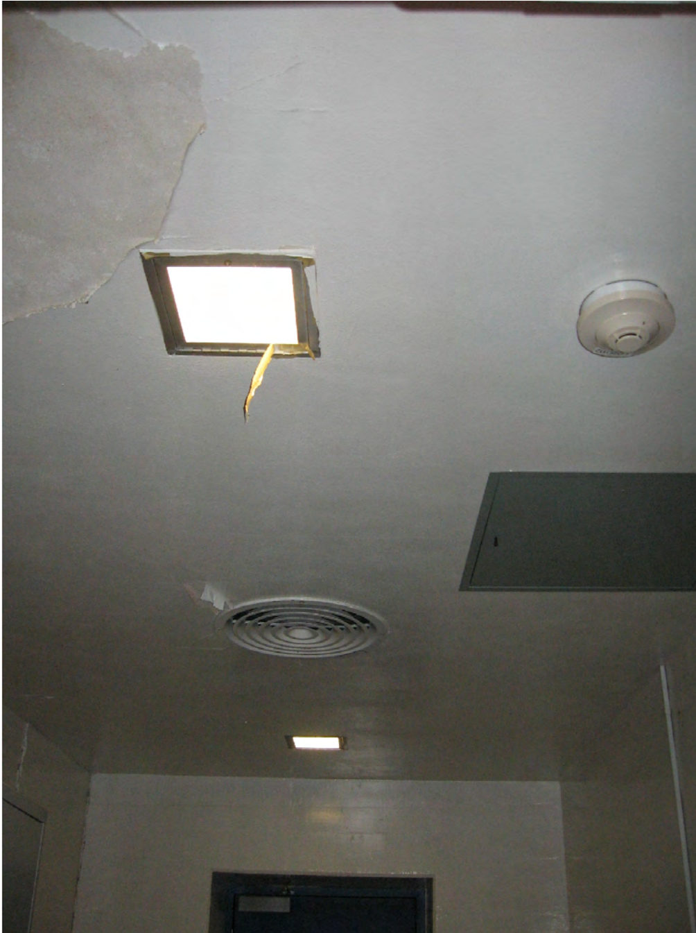
Figure 27: The new Avigilon security camera will be mounted at the ceiling just inside the northeast Powerhouse door entrance.
